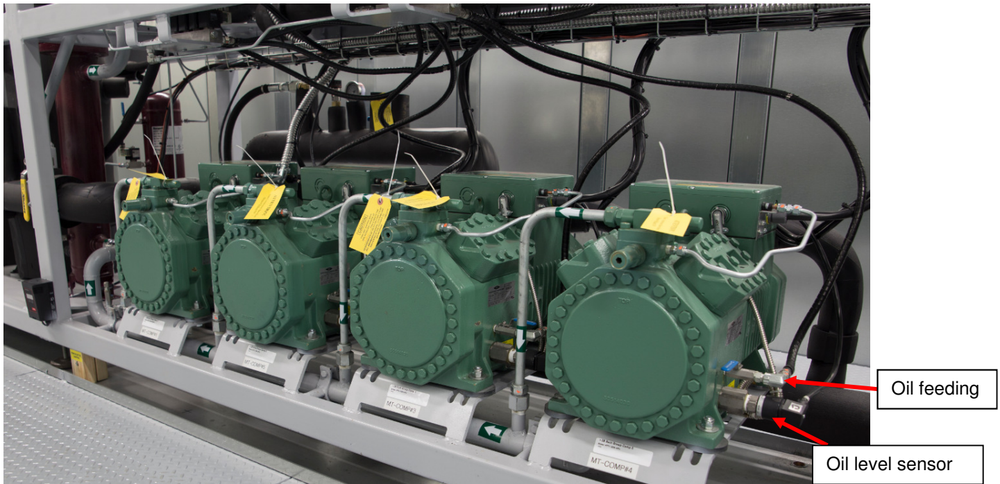
Figure 3. Example of electronic oil level regulators for CO 2 transcritical compressors applications.
