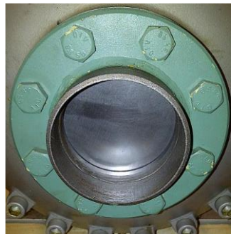
DN125 suction flange adapter
