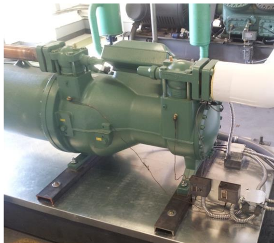
Installation of CS85 Shown
